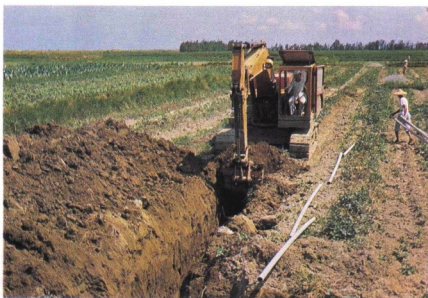
地下暗管排水系統改良鹽分地 A subsurface tile drainage system used for reclaiming saline land.
