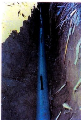
埋管 Pipe installation
