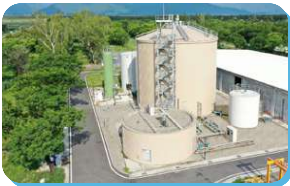
Biogas Center in the Park
