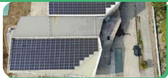
Roof-type solar PV (Yulin Huwei Rice Mill)
