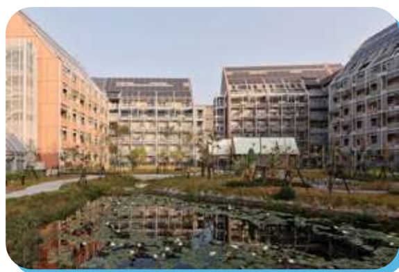
Shalun Smart Green Energy Circular Residential Park
