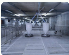
Comfortable pig housing with negative pressure ventilation and water curtain
