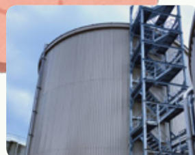
Renewable energy (biogas power generation)
